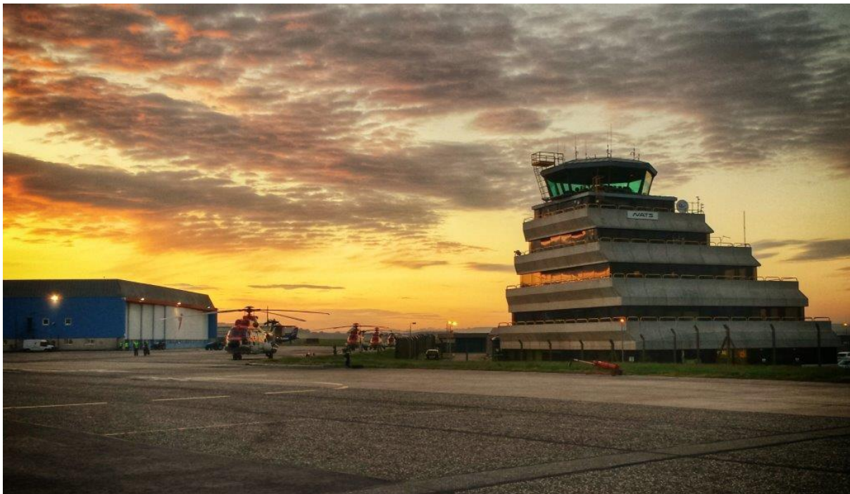
The NATS air traffic control tower at sunset
